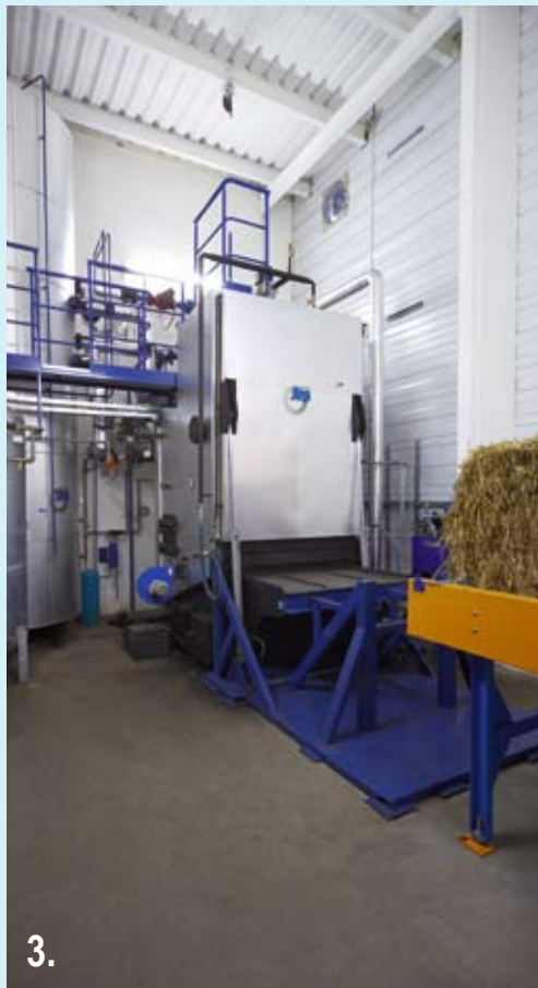
3. An example of one of the reference boiler plants for burning whole bales of straw, hay, flax, pressed paper boxes, etc., based at Step TRUTNOV. This boiler has received a „Gold Award“ from the Czech Building Academy and was rated the 2009 Best Building Product/Technology. (Tested under continuous measurement of emissions)
